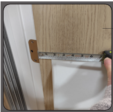
The space from the hinge side edge of the door to the edge of the space guard should not exceed 1 1/2"
